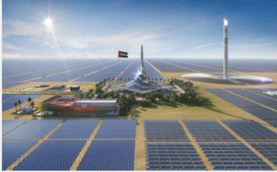
Source: Dubai commissions hydrogen plant
